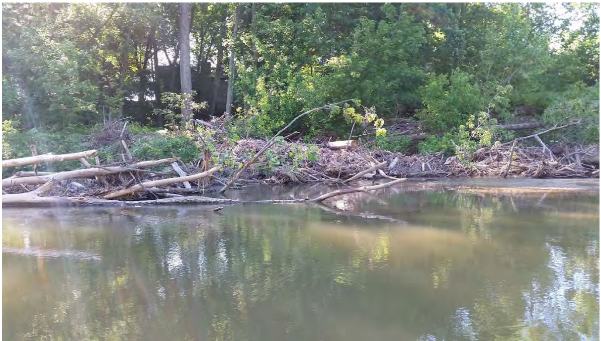
Photo 4: Debris along bank at FEH site
