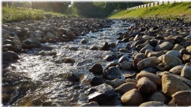
Figure 17: Armored Channel in Indianapolis, IN
