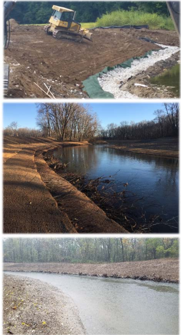
Figure 16: Toe Protection Measures Riprap toe protection (top); soil lifts above toe wood (middle); toe wood (bottom)
