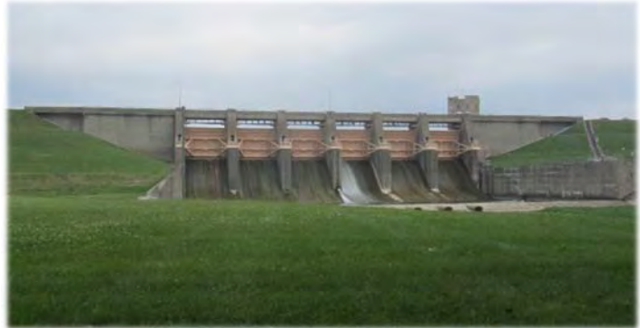
Figure 5: Eagle Creek Dam
