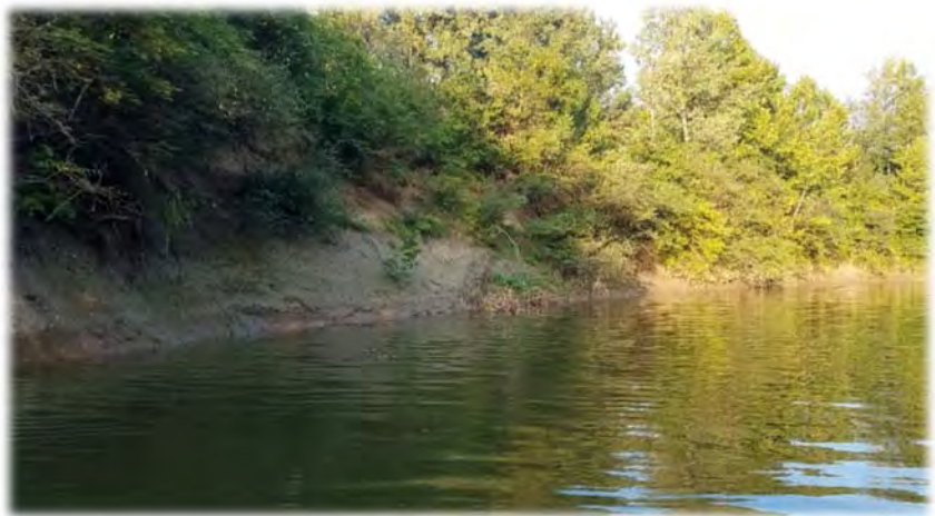
Figure 1: Stream Bank Along Eagle Creek Levee
