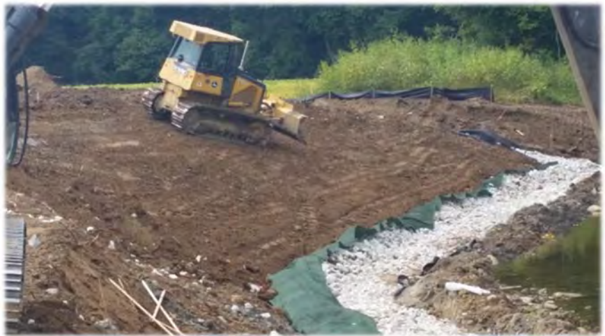
Figure 8: Toe Protection Measures
