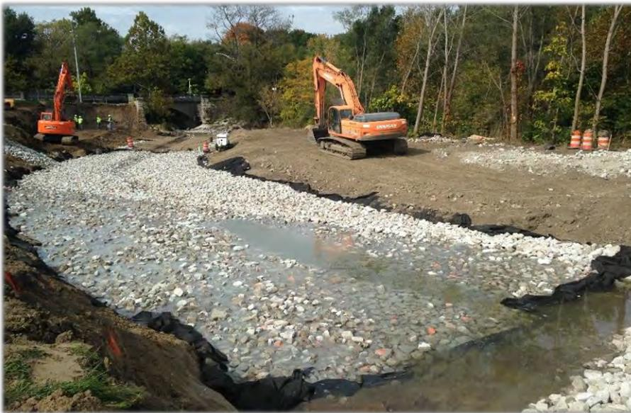
**Figure 4-28: Riprap Bed Armoring**
