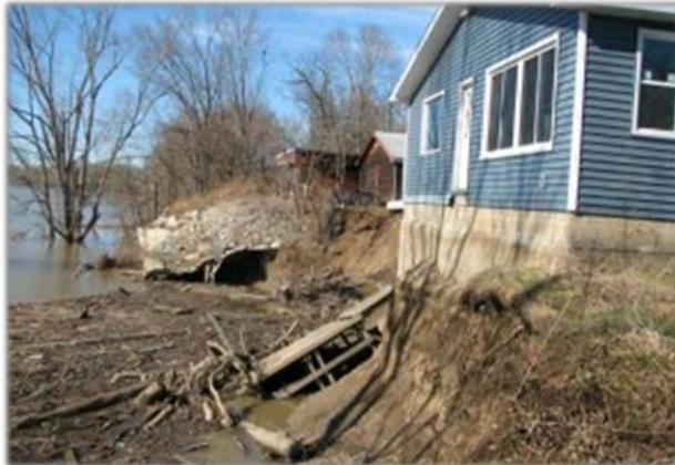
**Figure 1-1: Typical Example of a Fluvial Erosion Hazard**
