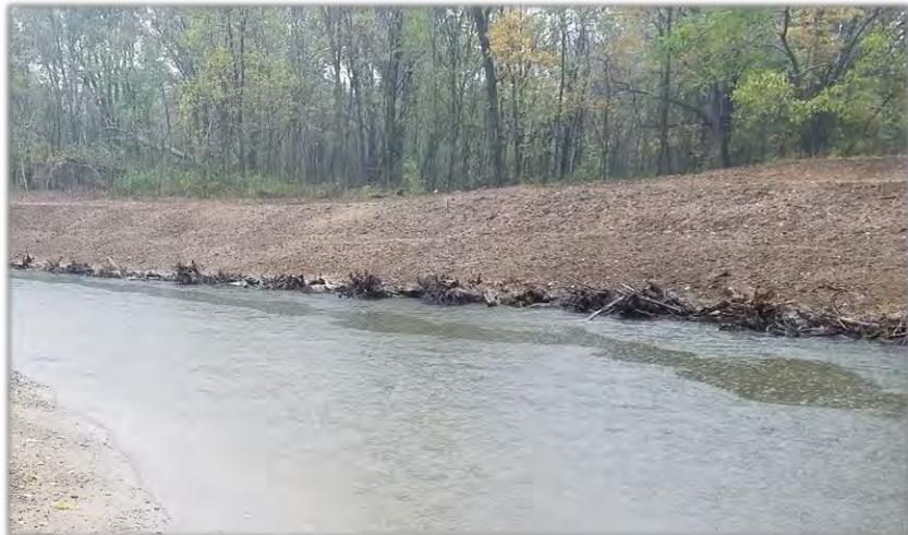
**Figure 4-30: Toe Protection – Toe Wood**
