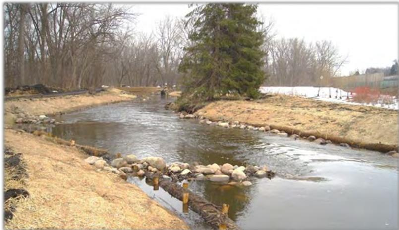
**Figure 4-32: Flow Redirection – Rock Vanes**
