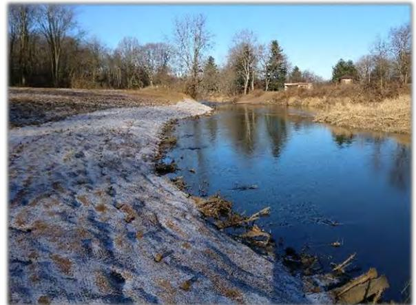
**Figure 4-40: Poor Vegetation Establishment Due to Unfavorable, Cold Weather**
