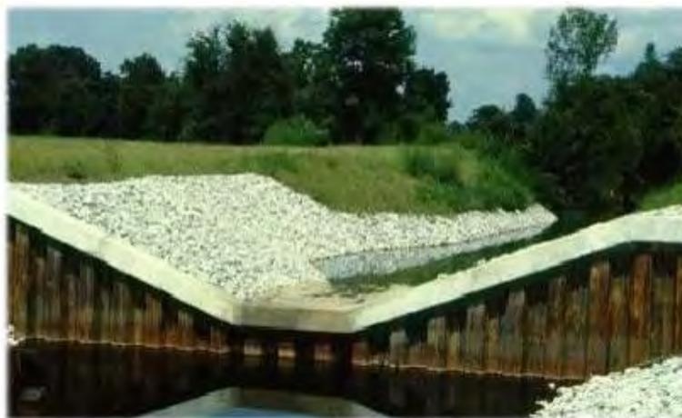
**Figure 4-27: Grade Control Structure**
