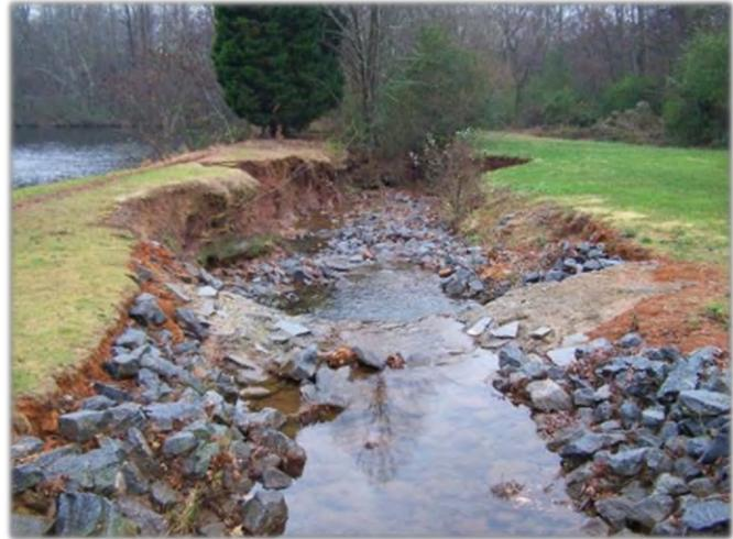
**Figure 4-9: Erosion Downstream of a Threshold Channel**
