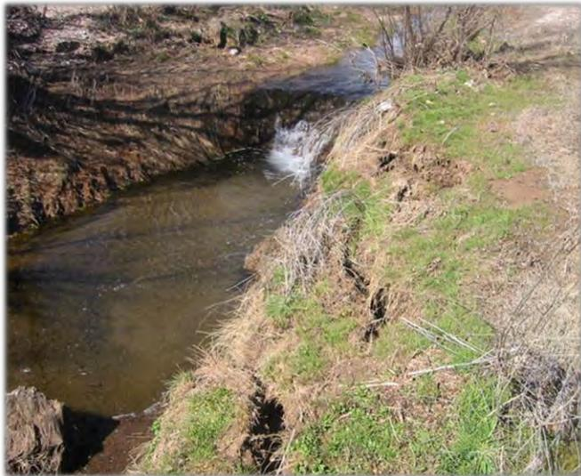
**Figure 4-24: Channel Experiencing Degradation via a Headcut**
